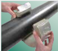
1. Ensure correct size of block. Lift sealing tag, open block and position around pipe.
