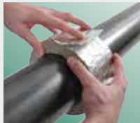
2. Close block around pipe and re-seal tag.
