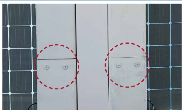
Hollo-Bolt (countersunk head) installed in a splice connection
