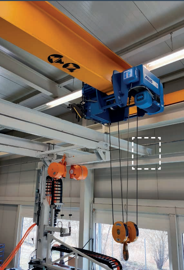
Photo shows additional steelwork and crane rails connected with Lindapter clamps to the existing frame of the production hall.
