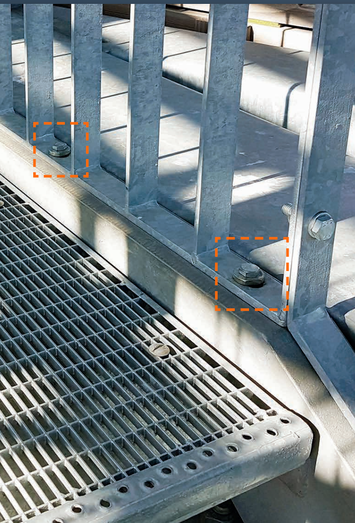
Photo shows railings connected to the structural hollow section of a staircase with Lindapter Hollo-Bolts.
