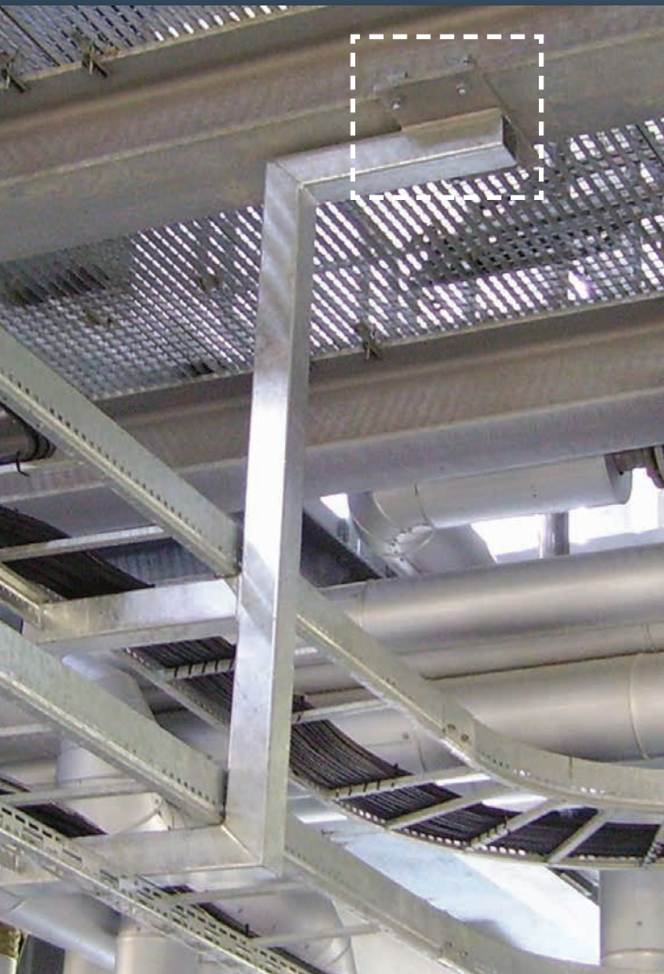
Photo shows a cable tray steel support arm connected to existing steel frame with Lindapter clamps.
