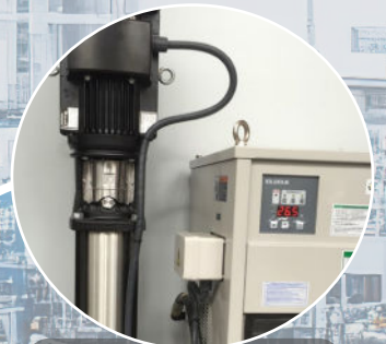
▲ Motors & Drives - Inside machinery
