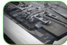
HVAC above carriage
