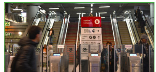
Lifts, Escalators & Lighting
