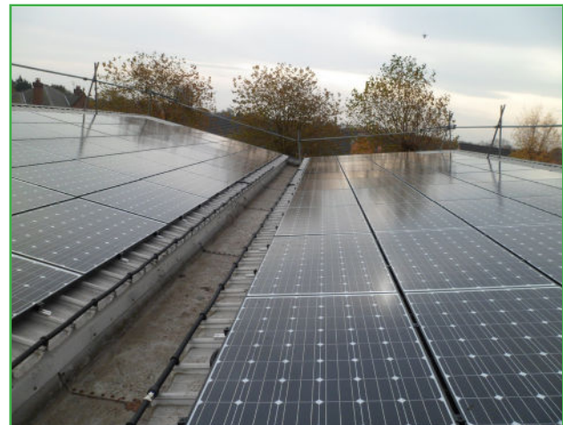
Atkore Flexicon Name: Liverpool Solar Vertical Market: Renewables Products Used: FPAS Conduit with FPA T-Pieces
